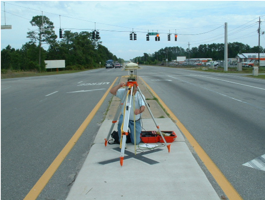
Figure 9-2. Static or Fast-Static survey techniques. Rover is set on a tripod accurately centered over a control point or feature such as a photo target. 5 minutes to 2 hours of static data may be collected whereas an RTK solution may have only a few seconds using a hand-held antenna pole.
