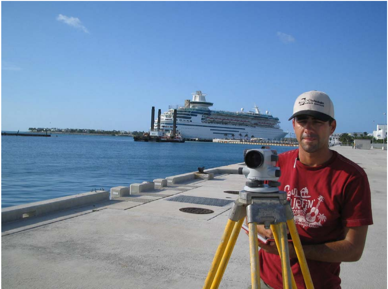
Figure 3-12. Sokkia B20 automatic level (Key West Harbor Dredging Project 2004-- C & C Technologies, Inc. & Jacksonville District)
