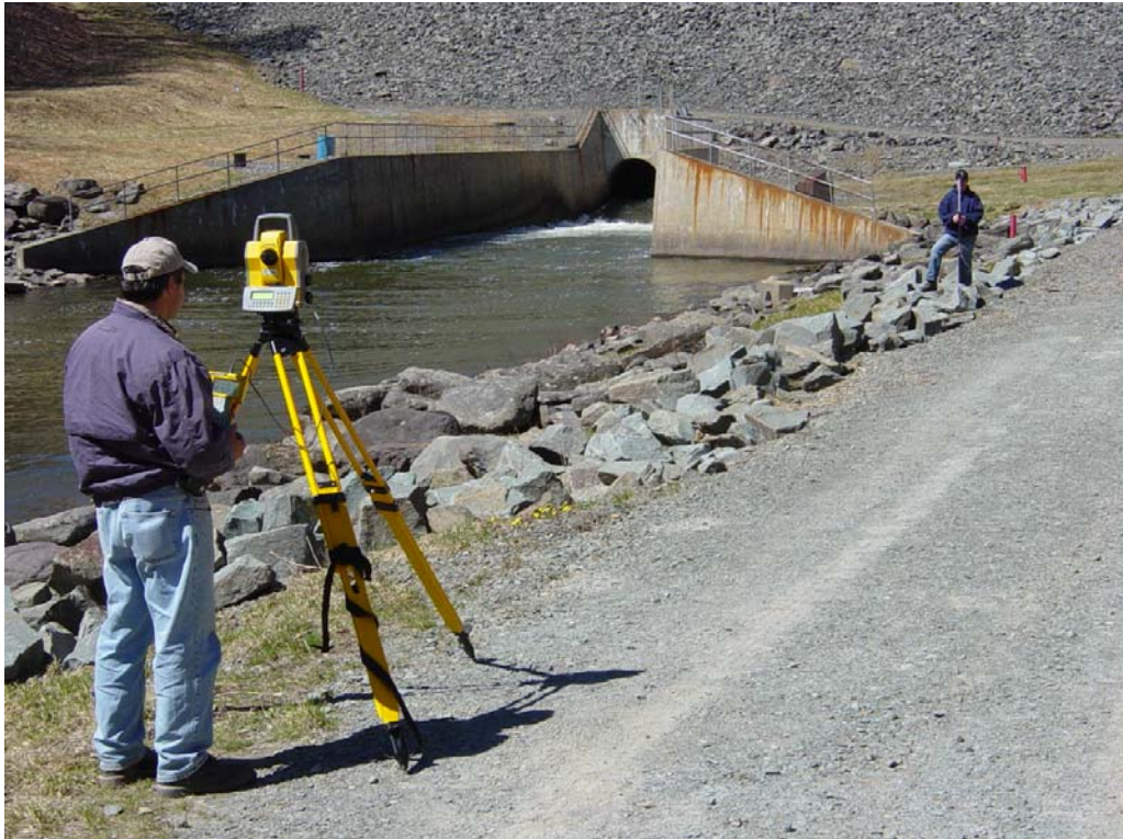
Figure 2-1. Topographic survey at Prompton Dam, PA (Philadelphia District--April 2005)
