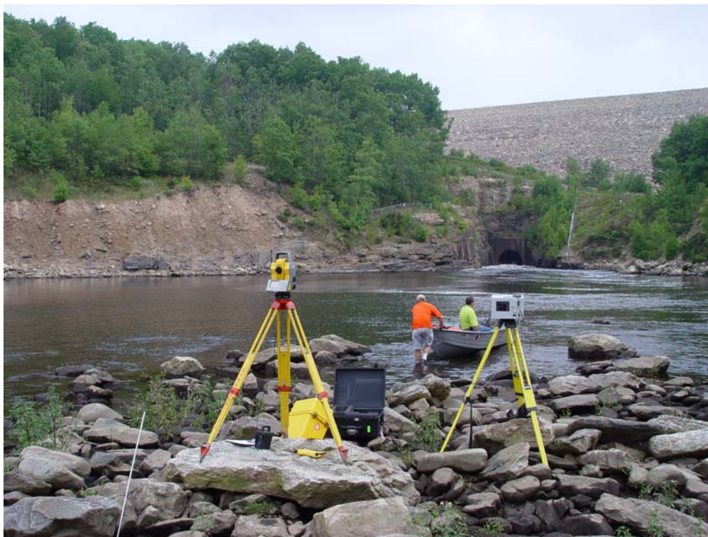
Figure 10-14. Reflectorless Total Station was utilized to georeference scanner data to project control network
