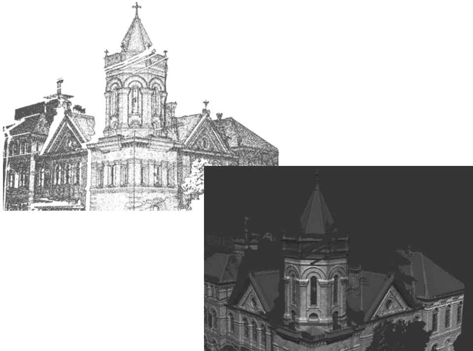
Figure 10-2. Laser scanned image (upper left) and rendered image (lower right) of Corps Mississippi River Division headquarters building, Vicksburg, MS (ARC Surveying & Mapping, Inc.)
