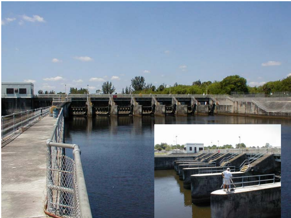
Figure 10-5. Typical scan location to cover downstream gate structures--instrument set up between 6th and 7th gates
