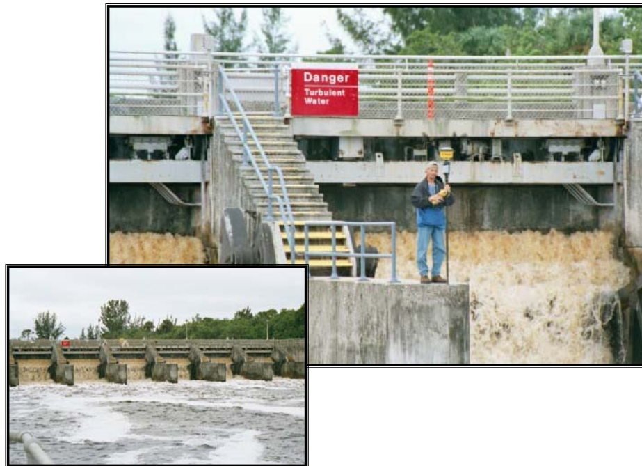
Figure 9-1. Real-Time kinematic survey of Corps lock and dam project--hand-held fixed height antenna pole
